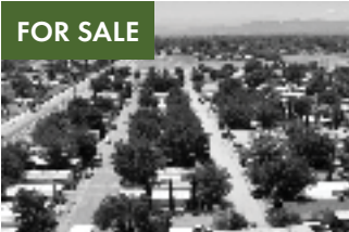
STABLE W/STRONG OCCUPANCY Lancaster, California
